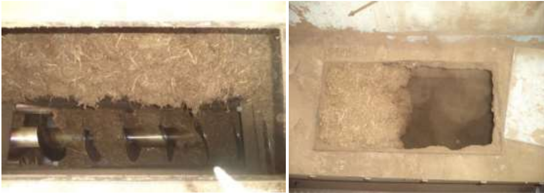
Figure: Blockages in screw conveyors.
